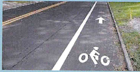
Separated bike lanes On-street or on-sholder marked bike lanes designate space for bicyclists. (5' to 6' wide)
