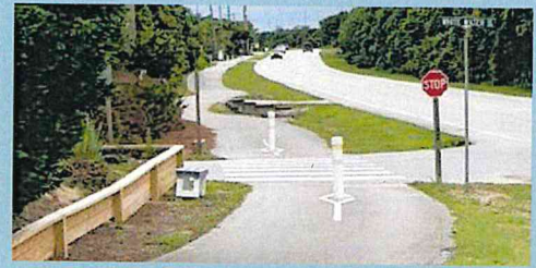
Separated multi-use paths A wide paved path for a bicyclists, pedestrians, runners, scooters, and others traveling for recreation or transportation. (8' to 12' wide)
