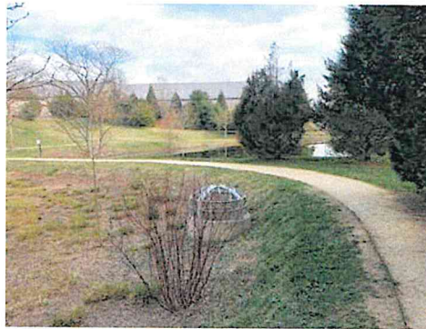
Recreation Example - Planted retention basins temporarily store runoff from parking areas. Overflow drains, like the one in the background of this image, divert water to the stormwater system if the basin fills.
