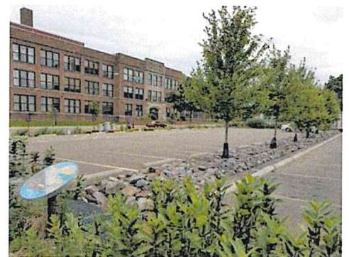
Development Example - Parking lot swales collect runoff from parking lots and direct the stormwater to a retention area. Planted swales and retention basins help to filter stormwater and prevent flooding.
