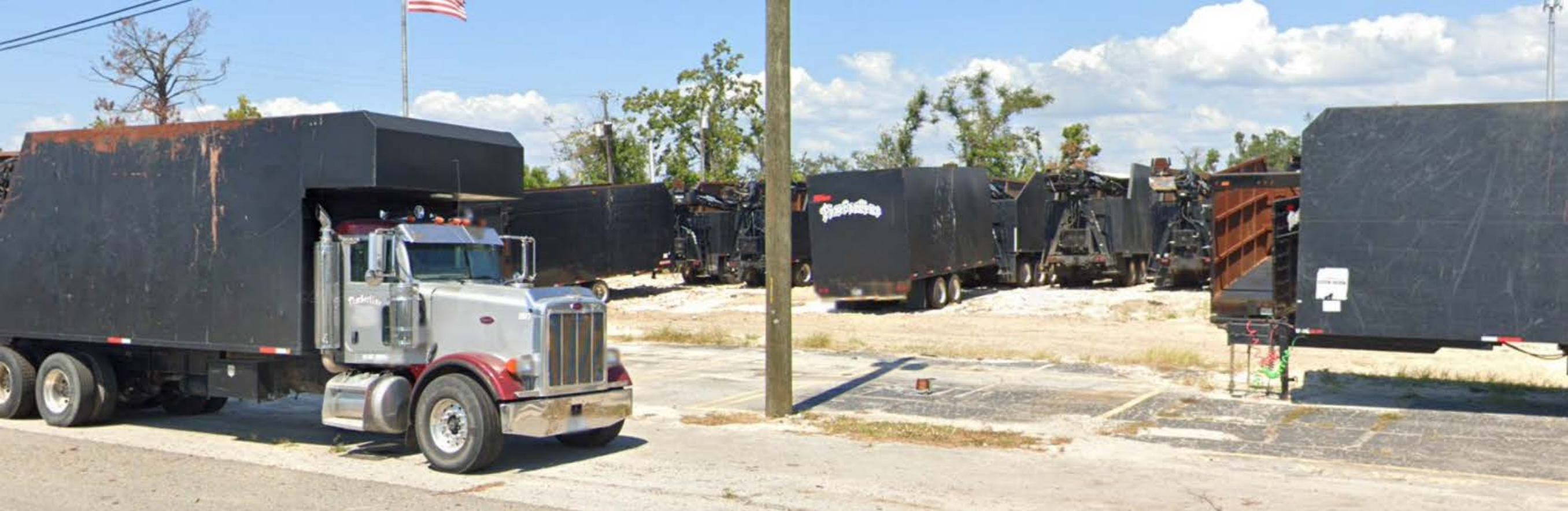
Building Replaced with Debris Trucks after Hurricane Michael took the building down
